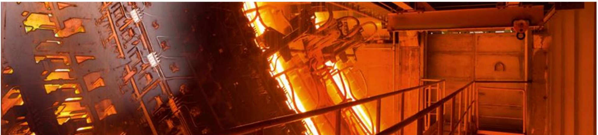
Dual Line lubrication System operating in a continuous casting environment
